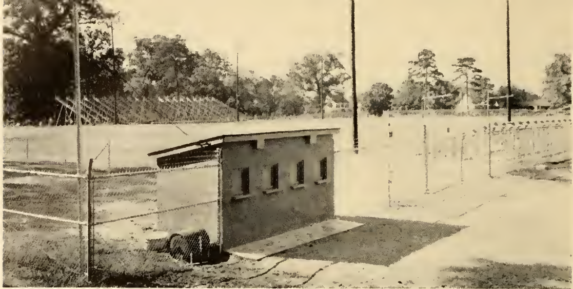
The new field with the bleachers next to the Woods incomplete. The houses seen in the background are on Court Street.
